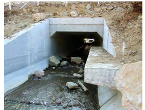
Figure 3-91 | Culvert with high-water ledge for small mammal crossing
