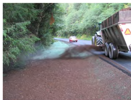
Figure 5-24 | A manure spreader adapted to side cast shredded wood
