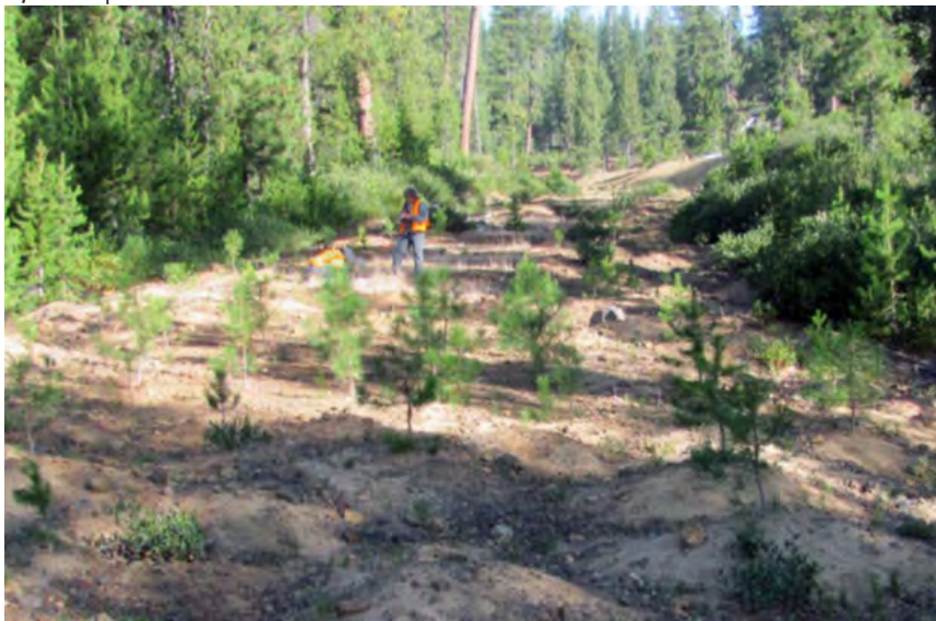
Figure 1-2 | Recently planted trees on an obliterated section of highway in Oregon
