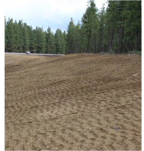
Figure 5-13 | Trackwalking compacts soils
