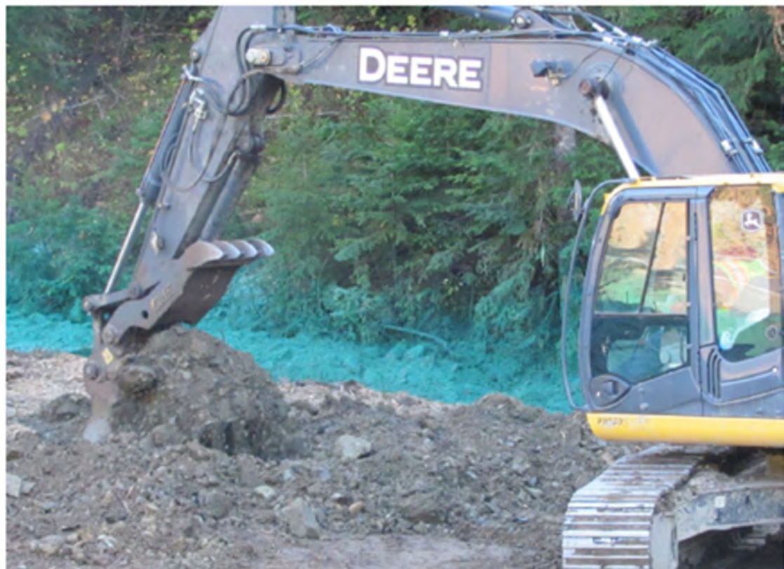
Figure 5-12 | Excavators decompacts and incorporates soil amendments
