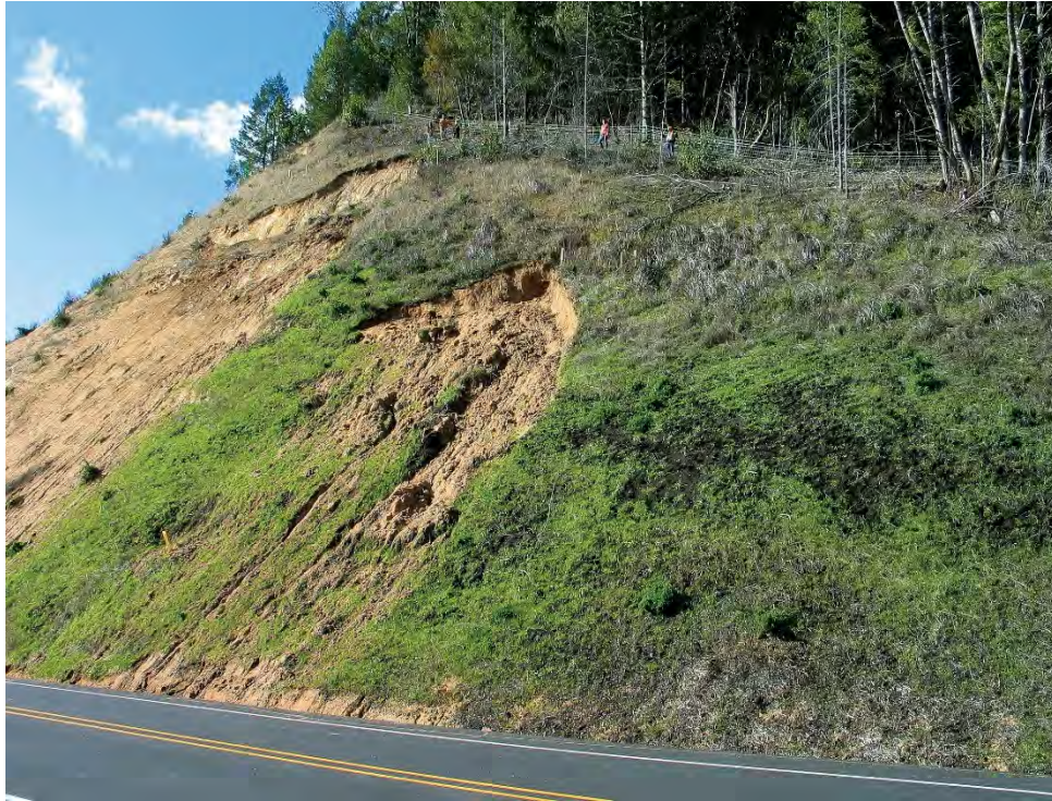
Figure 3-72 | Effects of roots on slope stability
