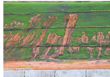
Figure 3-68 | Restrictive layers can decrease slope stability
