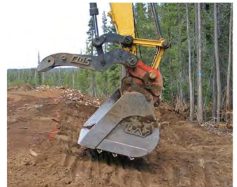
Figure 5-14 | Soil imprinting with modified excavator bucket
