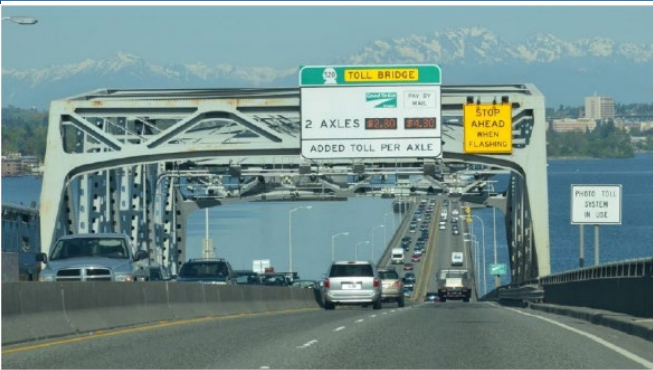
Credit: Washington State Department of Transportation
