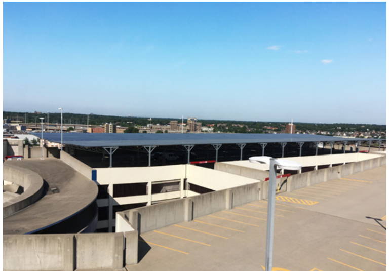
Figure 4: A rooftop solar garden on the ABC Ramps Mobility Hub in downtown Minneapolis. Source: MnDOT
