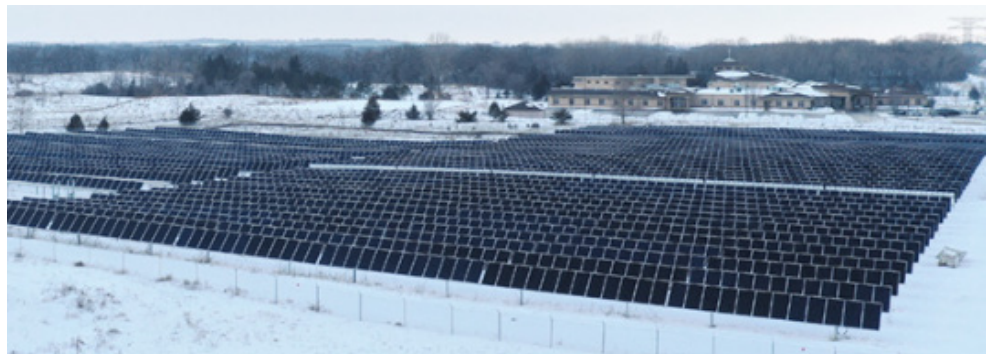
Figure 5: A 1-megawatt community solar garden in Afton, MN, formerly a gravel pit. Source: MnDOT
