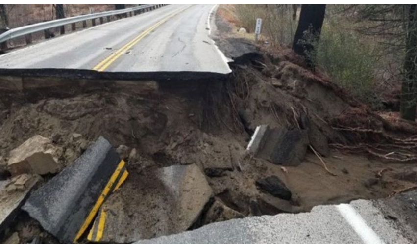
When soil erosion starts occurring it can get progressively worse and start to erode the soil under the road causing roadway collapse.
