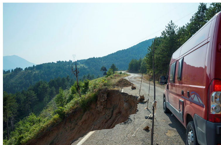
When soil erosion starts occurring it can get progressively worse and start to erode the soil under the road causing roadway collapse.
