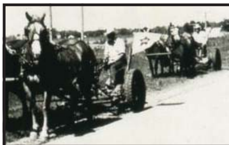
In the 30s, mowing was reported to cost 50 cents per lane mile. Savings were found by attaching the blade to a truck.
